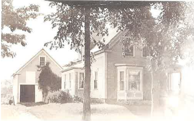
Above, as the house appeared in early 1900s. To the right, as it appears today.
